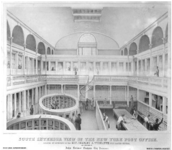
Thompson's New York City Post Office
