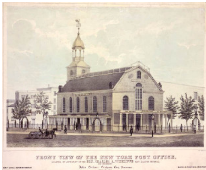
Thompson's New York City Post Office
