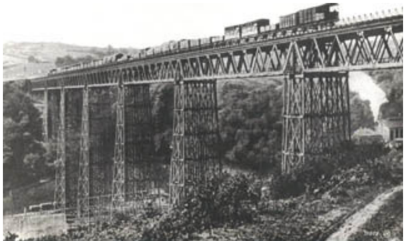
The Crumlin Viaduct -One of the great technological triumphs of early Victorian England.
