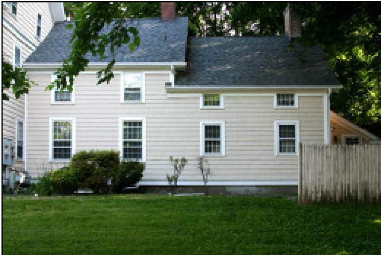
The eastern wing of the Coles homestead (on the right) is the oldest part of the house.
